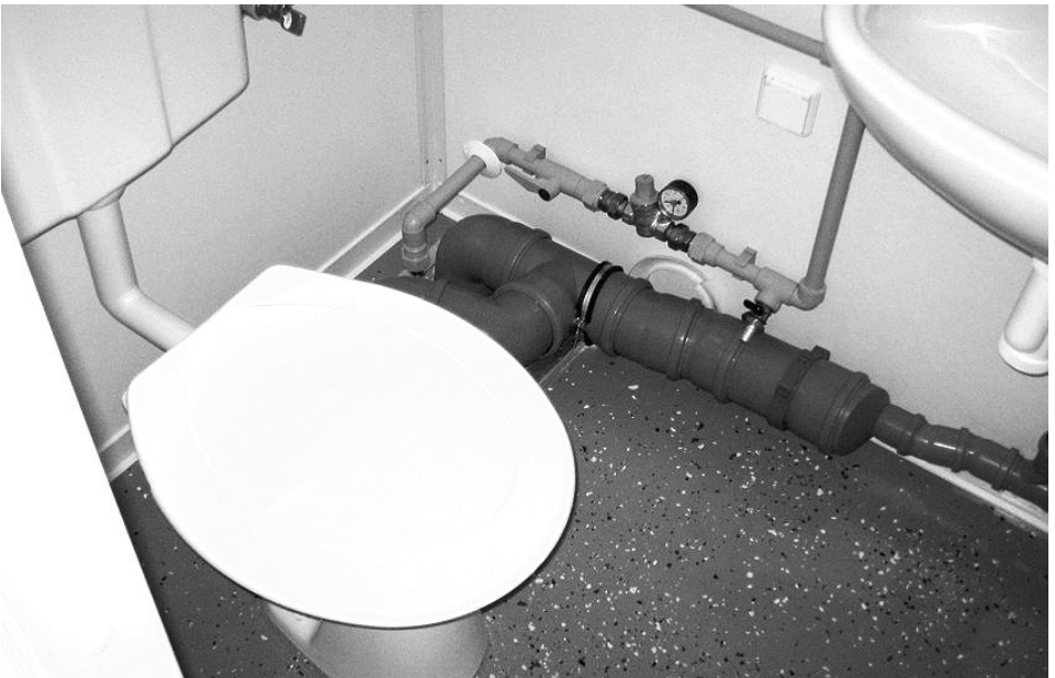
Figure 12 Installing through the floor
