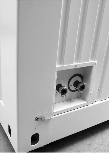
Figure 11 Water supply and sewage line outlet through module side wall
