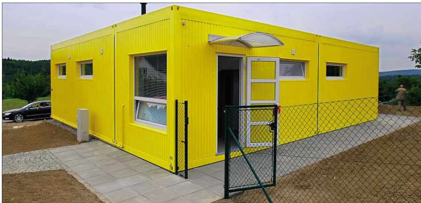
FOTO: KOMA MODULAR CONSTRUCTION
